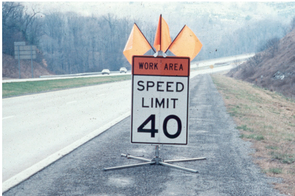
Figure 3.3.4 Work Area Speed Limit Sign (Regulatory)
