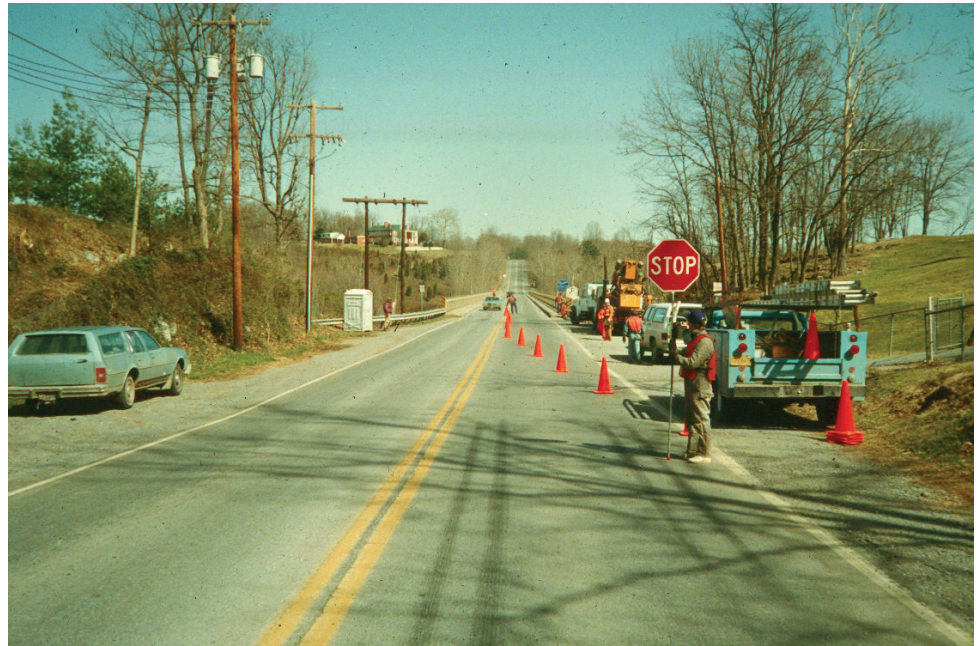
Figure 3.1.4 Traffic Control Operation
