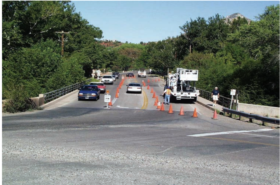
Figure 3.3.1 Traffic Control Operation
