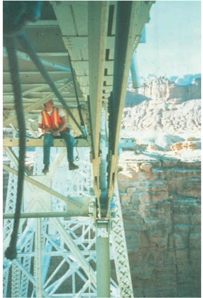
Figure 3.5.4 Rigging for Superstructure Inspection
