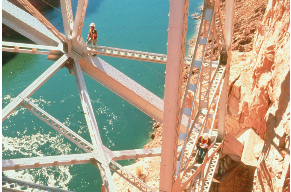
Figure 3.2.7 Inspection Involving Extensive Climbing
